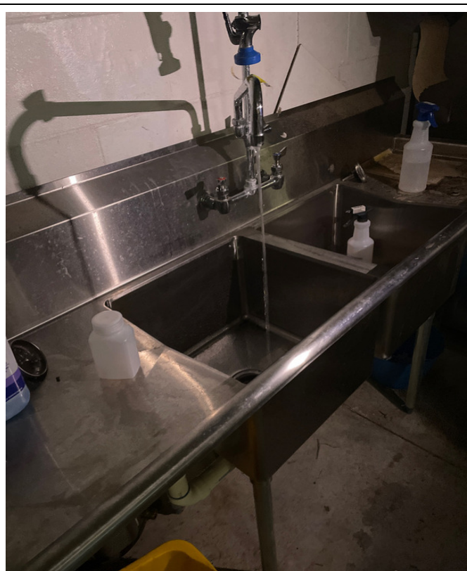
100-2 - AG Building - Shop South Wall
