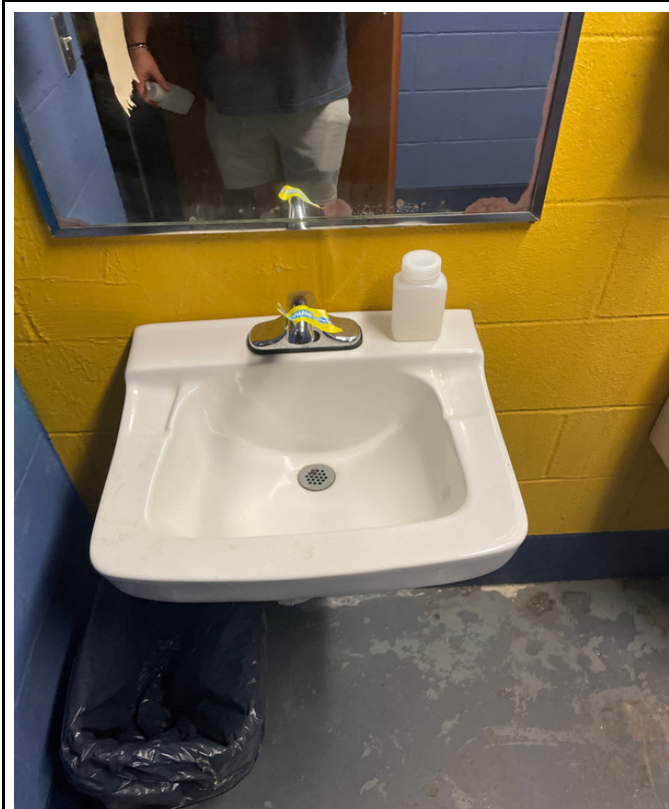
100-3 - AG Building - Shop Men's Restroom
