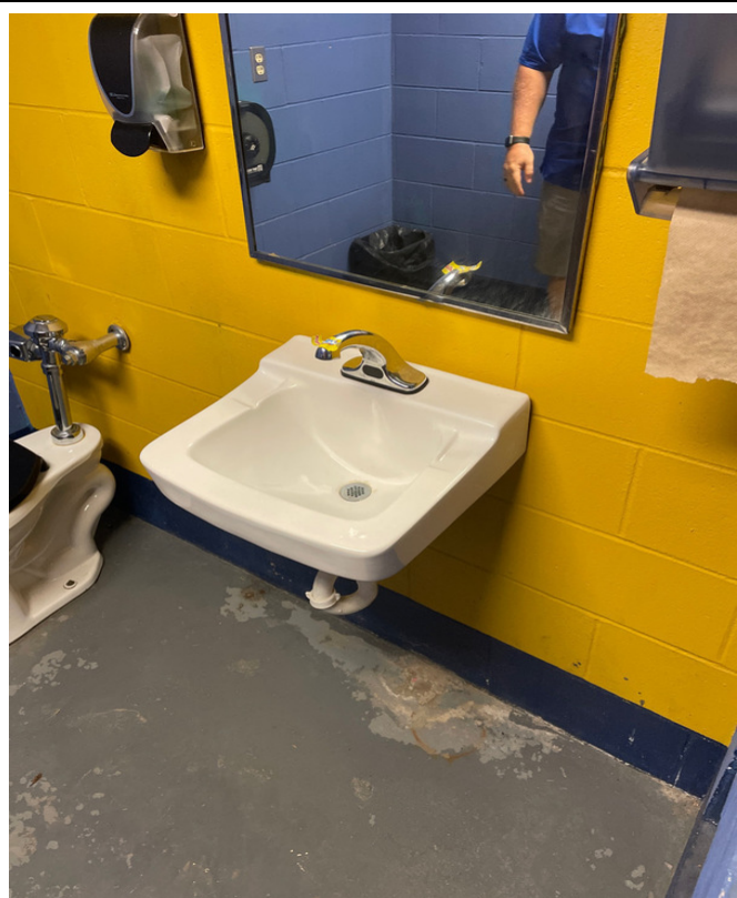
100-4 - AG Building - Shop Women's Restroom
